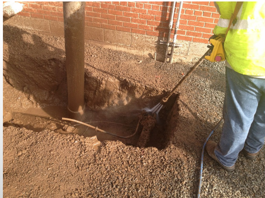
Hydrovac excavation
