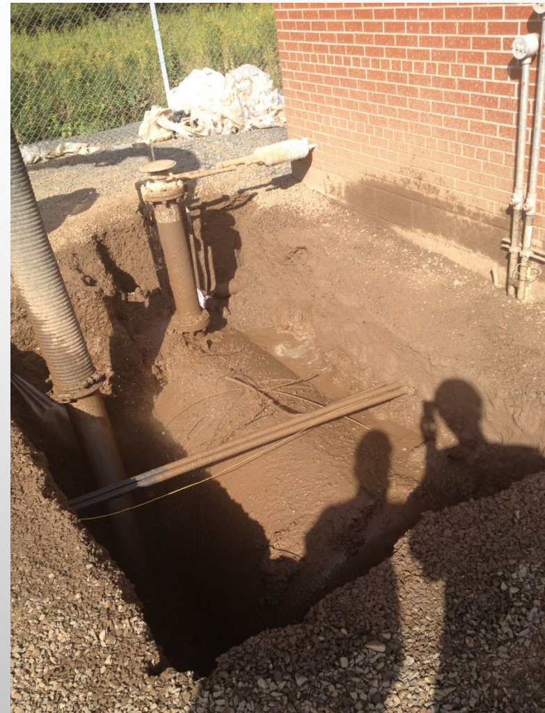
Hydrovac excavation
