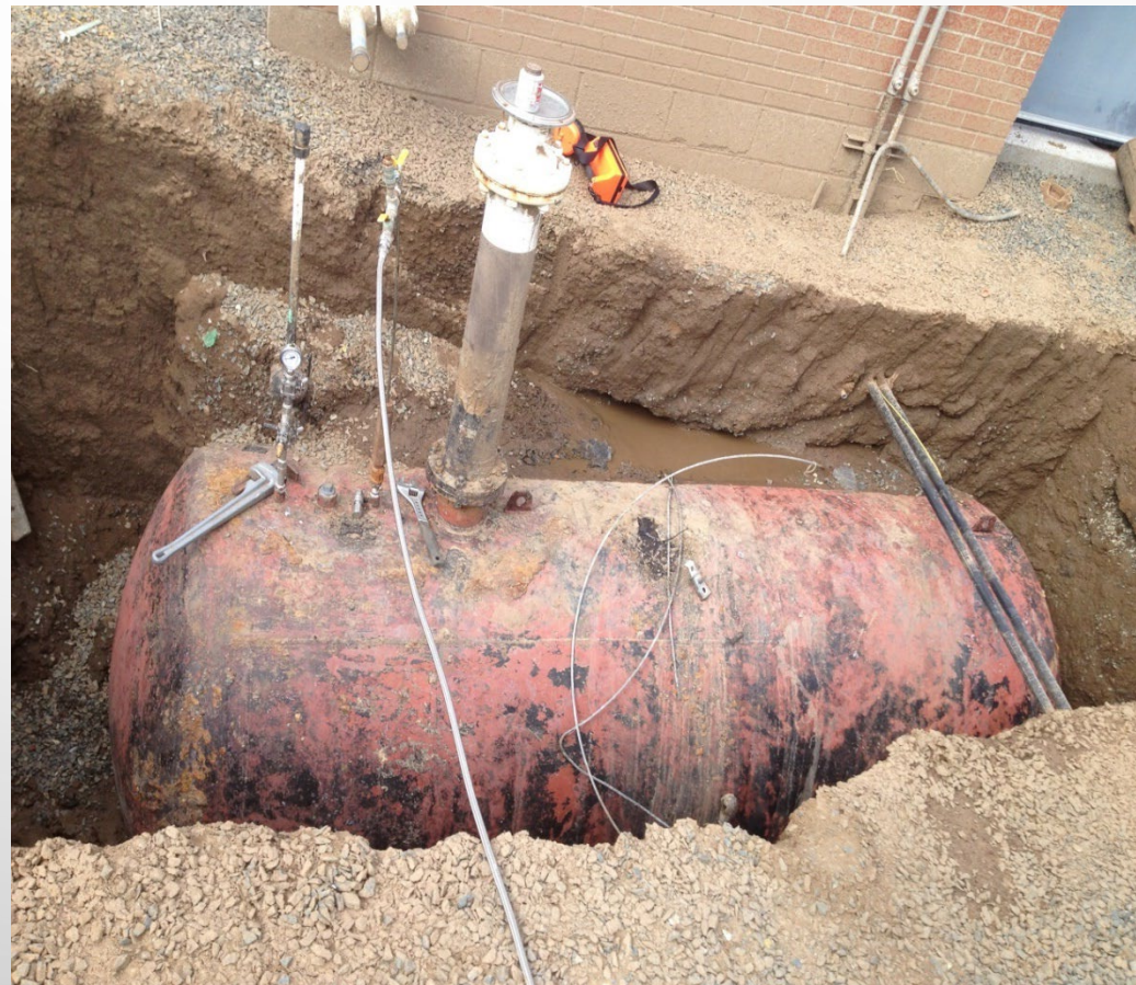
Draining odorant from the tank
